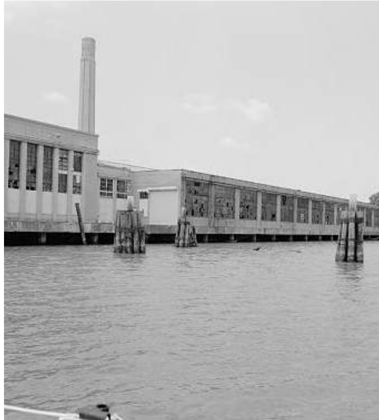
Demolished Ford Plant/ Waterfront Industrial History
