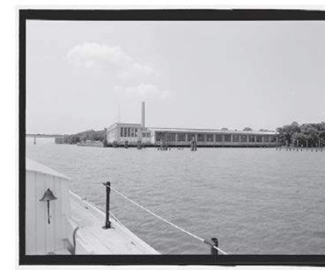
11. DEMOLISHED FORD FACTORY
