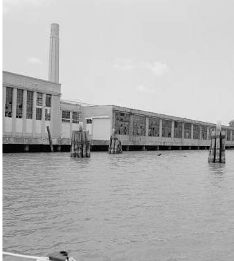
Demolished Ford Plant/ Waterfront Industrial History
