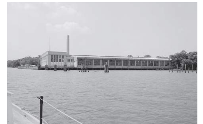
12. DEMOLISHED FORD FACTORY
