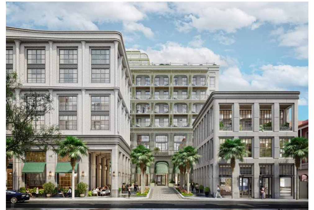
Four Seasons Hotel & Residences, Charleston, SC
