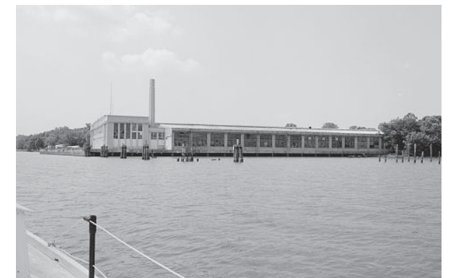
12. DEMOLISHED FORD FACTORY
