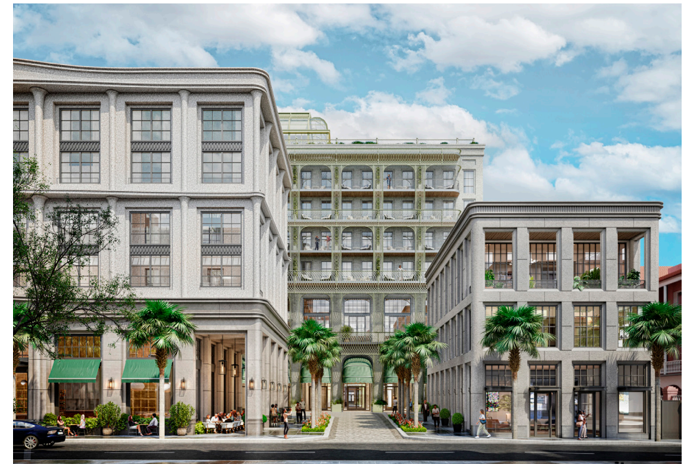
Four Seasons Hotel & Residences, Charleston, SC
