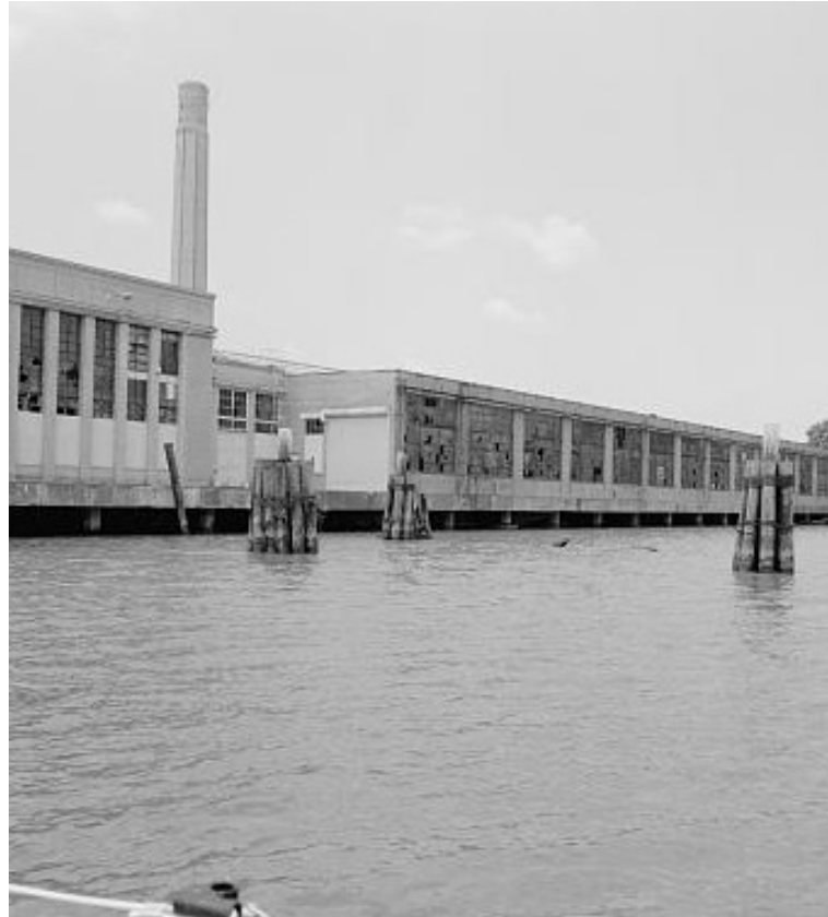
Demolished Ford Plant/ Waterfront Industrial History
