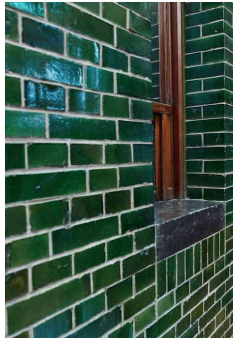
GLAZED BRICK/TILE LOGGIA
