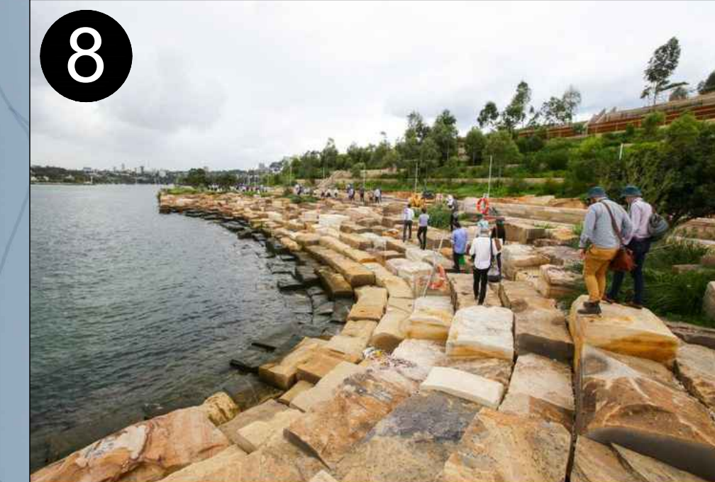
8 BLOCK SEATING AND SHORELINE STABILIZATION
