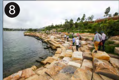
BLOCK SEATING AND SHORELINE STABILIZATION
