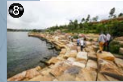
BLOCK SEATING AND SHORELINE STABILIZATION
