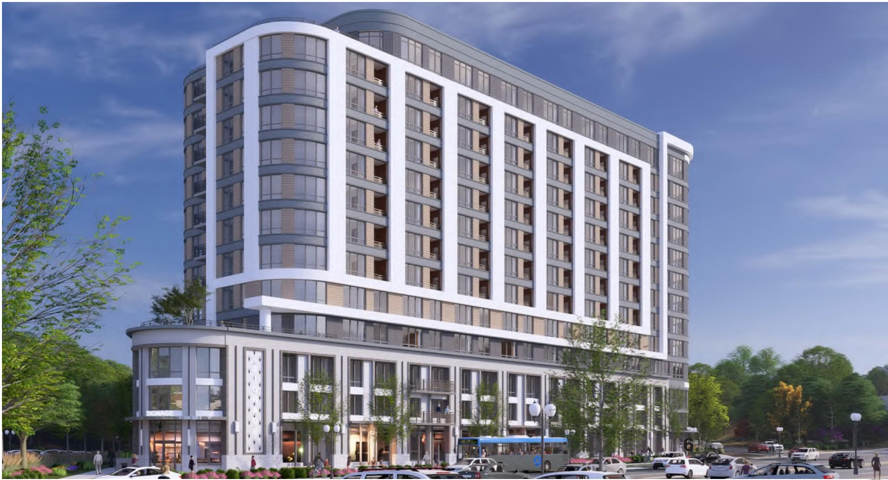
VIEW FROM NORTHEAST AT LANGSTON BLVD
