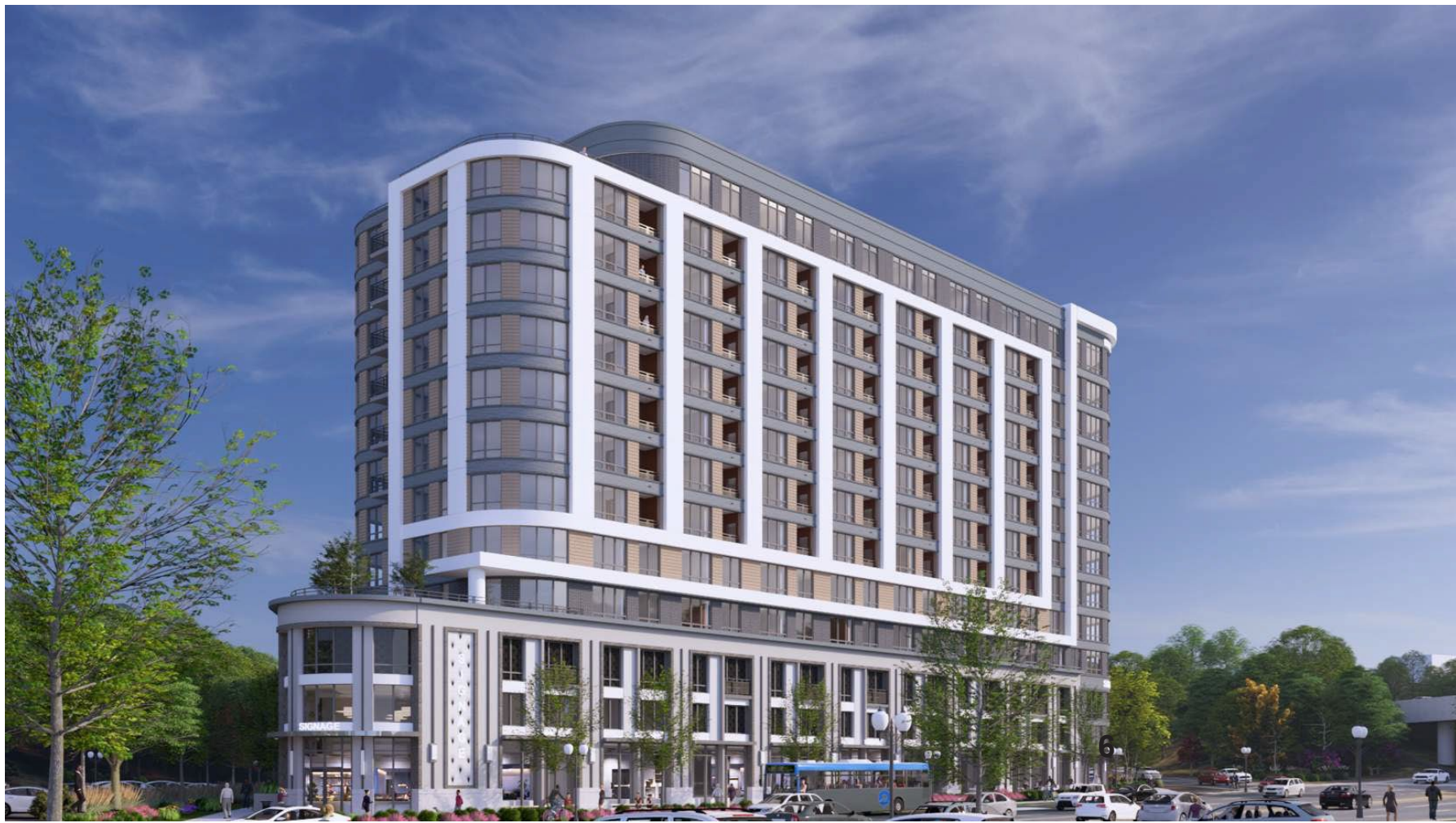
VIEW FROM NORTHEAST AT LANGSTON BLVD
