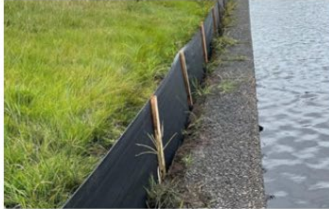
Erosion and sediment controls (silt fencing)
