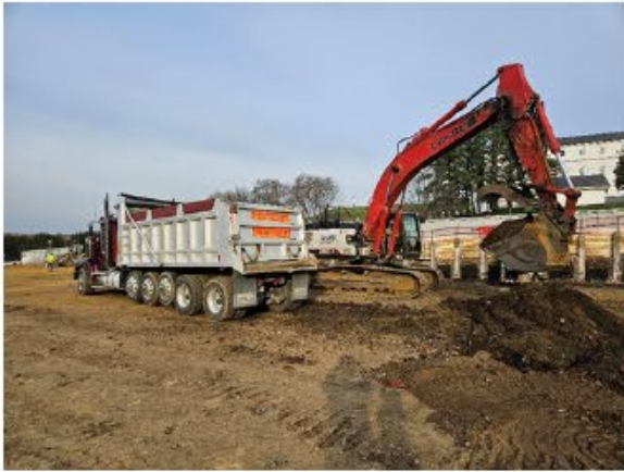
Direct loading of soil
