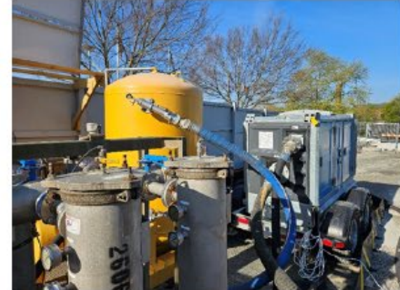
Water treatment before discharge
