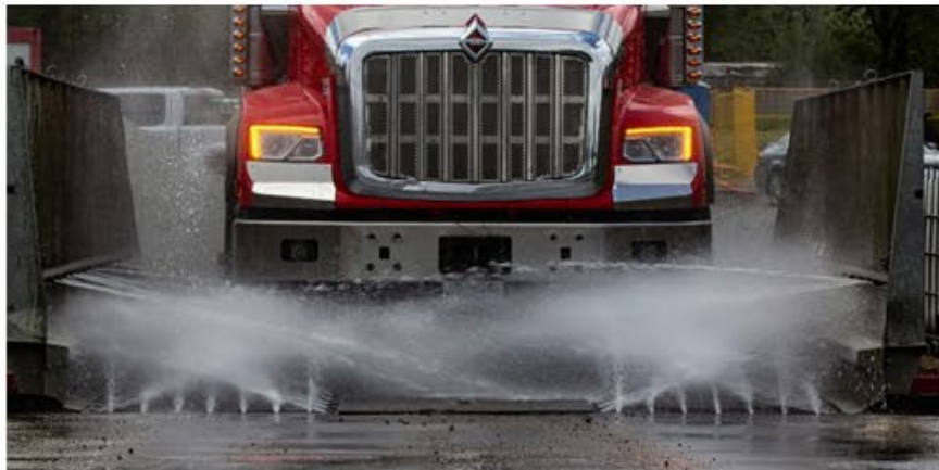
Wheel washing before exiting site
